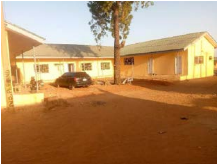
NVRI Zonal Laboratory left view under renovations
