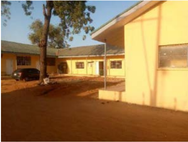
NVRI Zonal Laboratory right view under renovations
